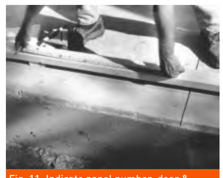
Fig. 11: Indicate panel number, door & windows openings, mechanical opening, etc.
