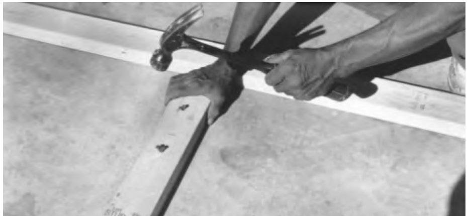
Fig. 8: Place cleats every 4 ft. and perpendicular to wall lines. (secure cleats with masonry screws Hilti, ITW Tapcon or similar).
