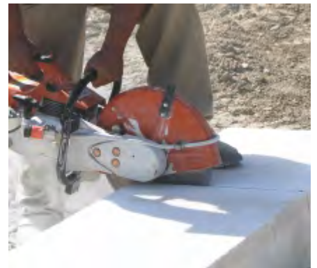
Fig. 25: Cut panels using a gasoline-powered circular saw.
