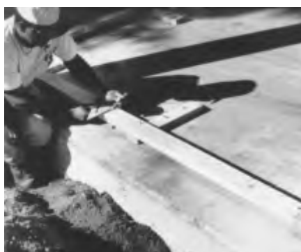
Fig. 10: Identify openings on template.
